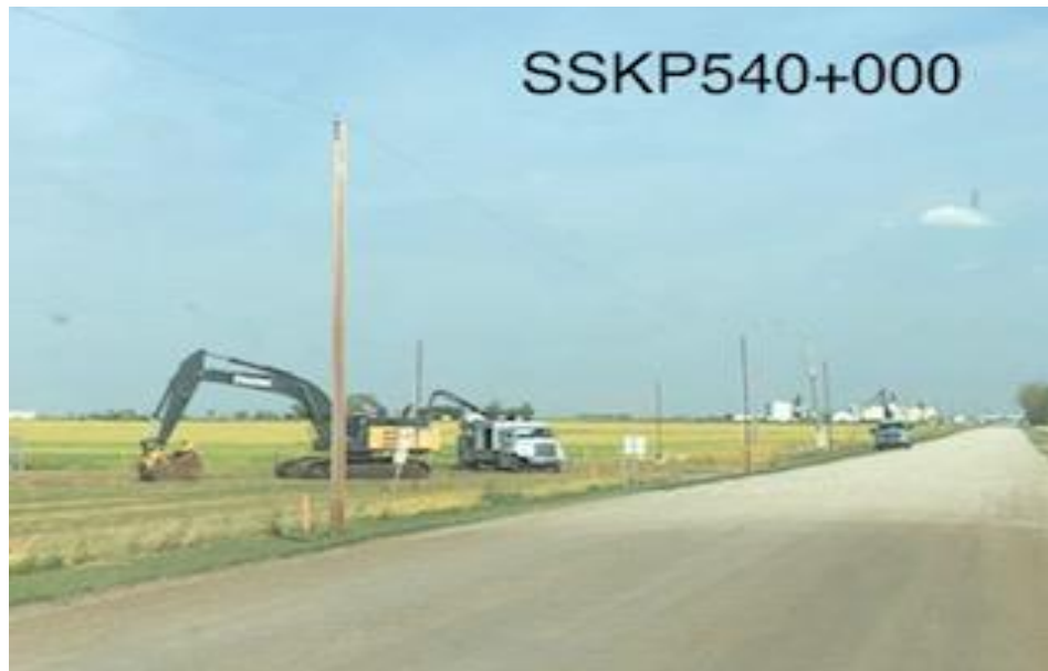
Hydro vac trucks daylighting underground lines
